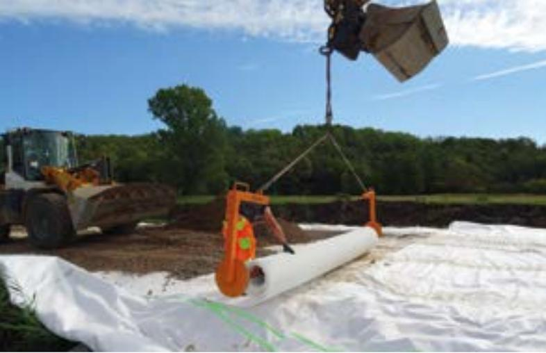
Fig. 1: Installation of Secugrid® HS by means of a spreader bar
