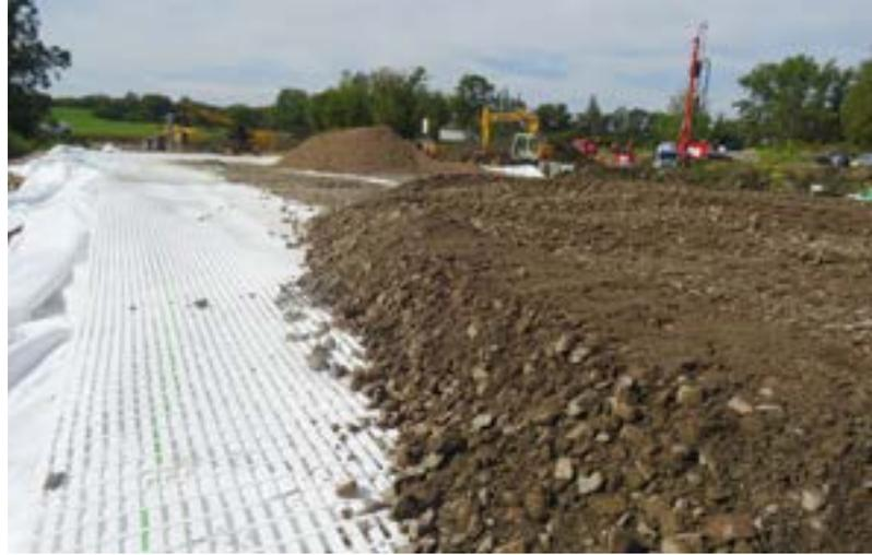
Fig. 2: Coverage with fill material
