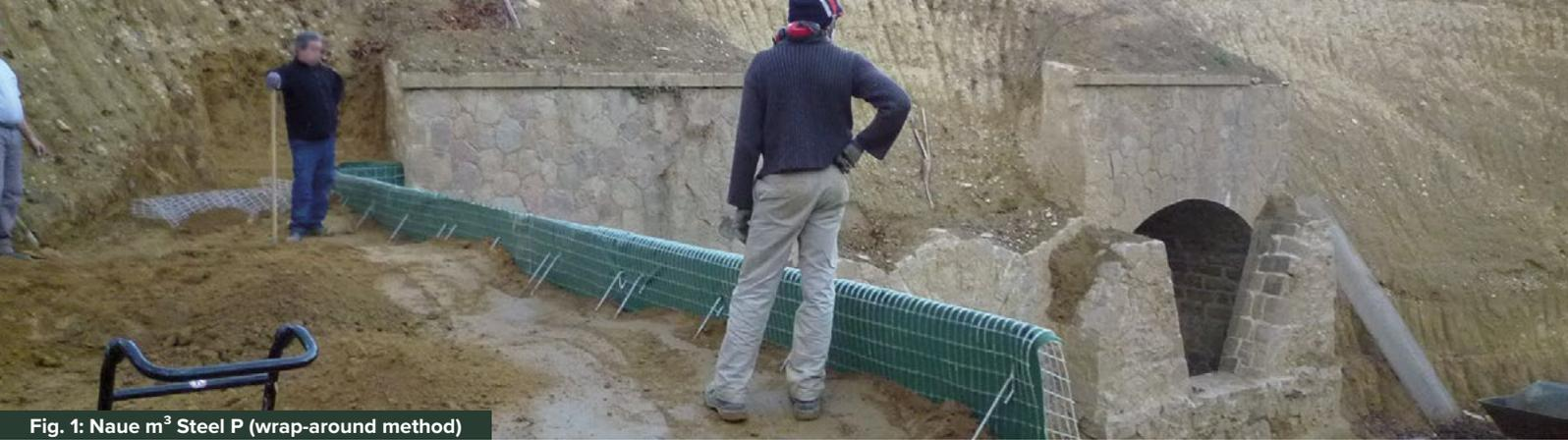
Fig. 1: Naue m<sup>3</sup> Steel P (wrap-around method)
