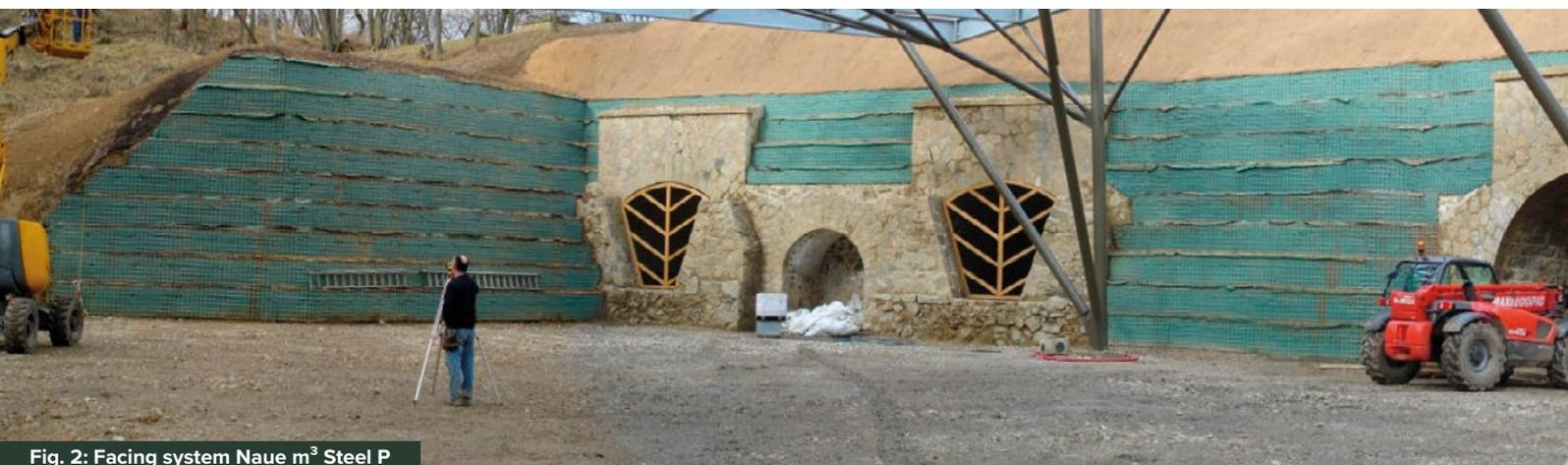
Fig. 2: Facing system Naue m<sup>3</sup> Steel P
