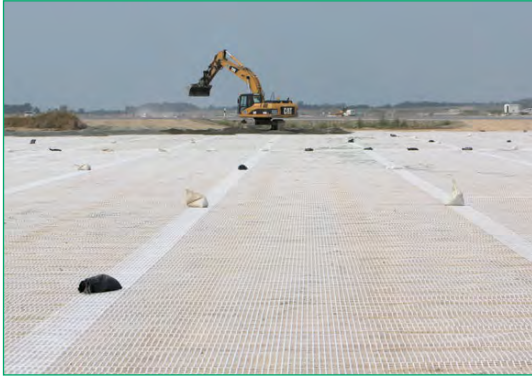
Fig. 7 Installed Secugrid® as a base course reinforcement
