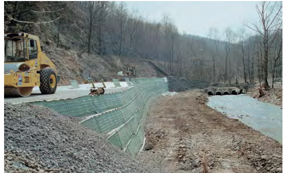
Railroad slope stabilisation
