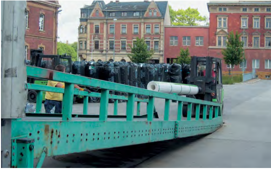
Loading of Secugrid®
