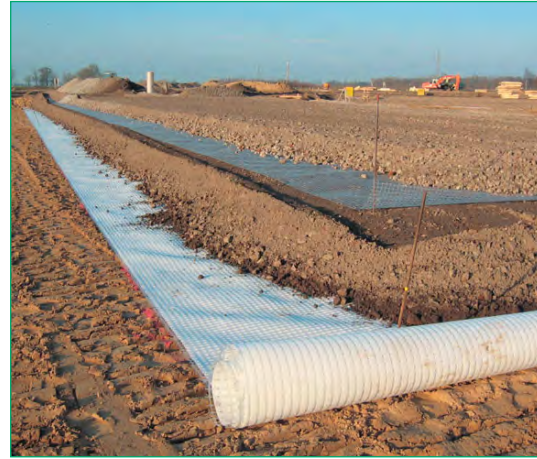
Fig. 8 Base course reinforcement on a very soft subsoil with Combigrid® (bottom) and Secugrid®
