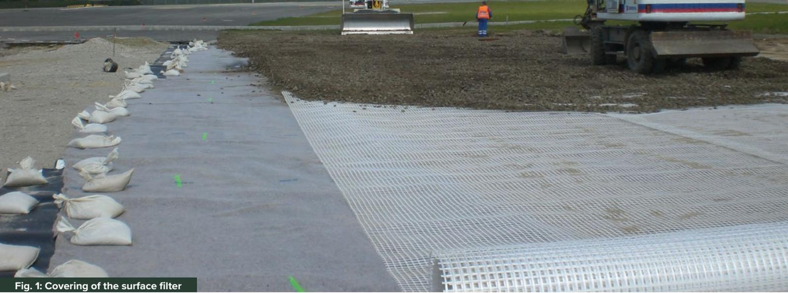
**Fig. 1: Covering of the surface filter**
