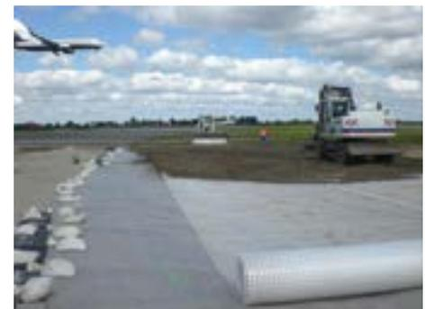
Fig. 3: Covering of the surface filter
