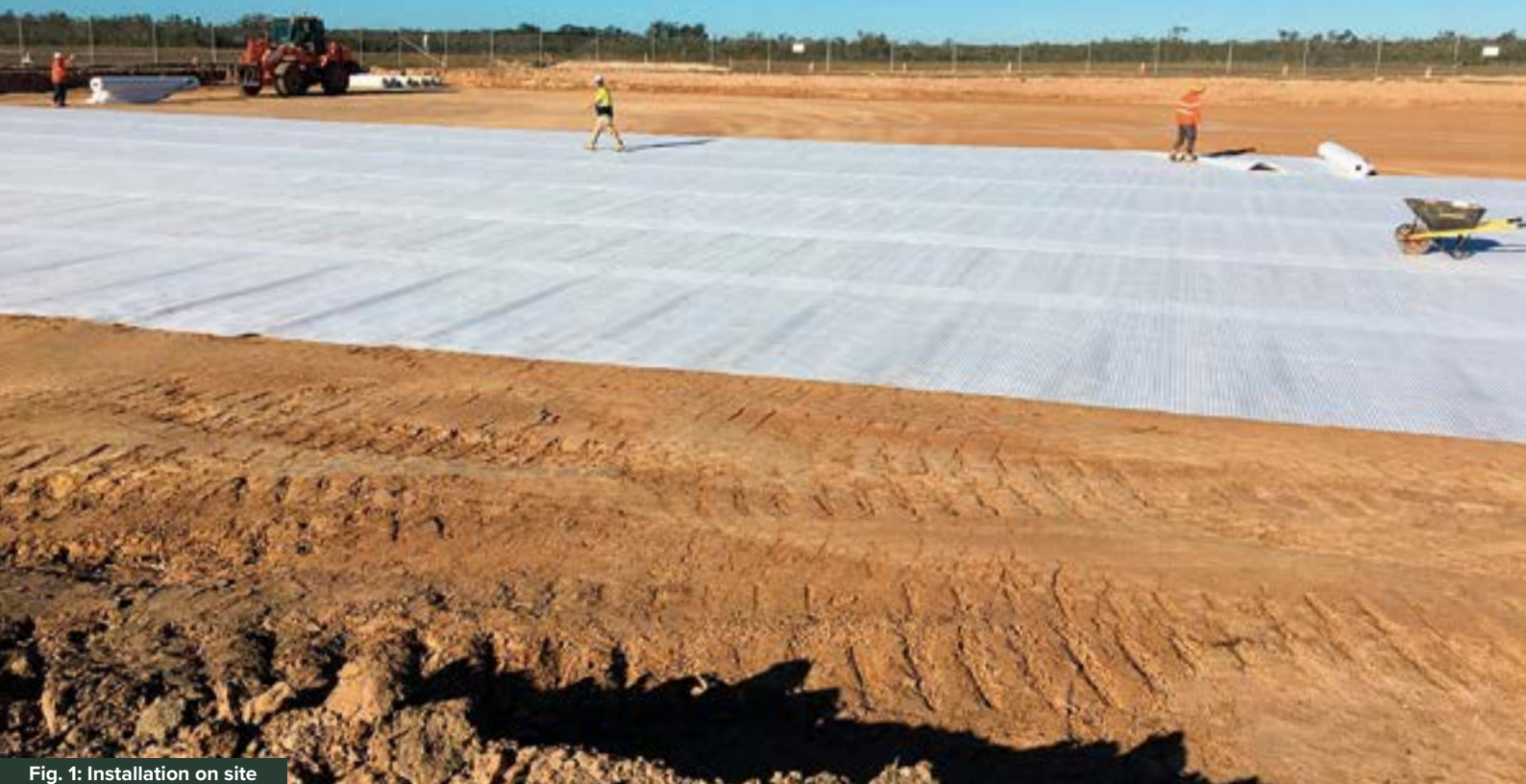
Fig. 1: Installation on site
