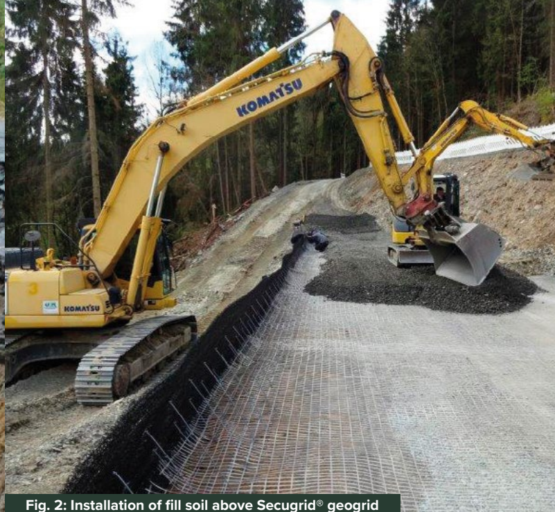
Fig. 2: Installation of fill soil above Secugrid® geogrid
