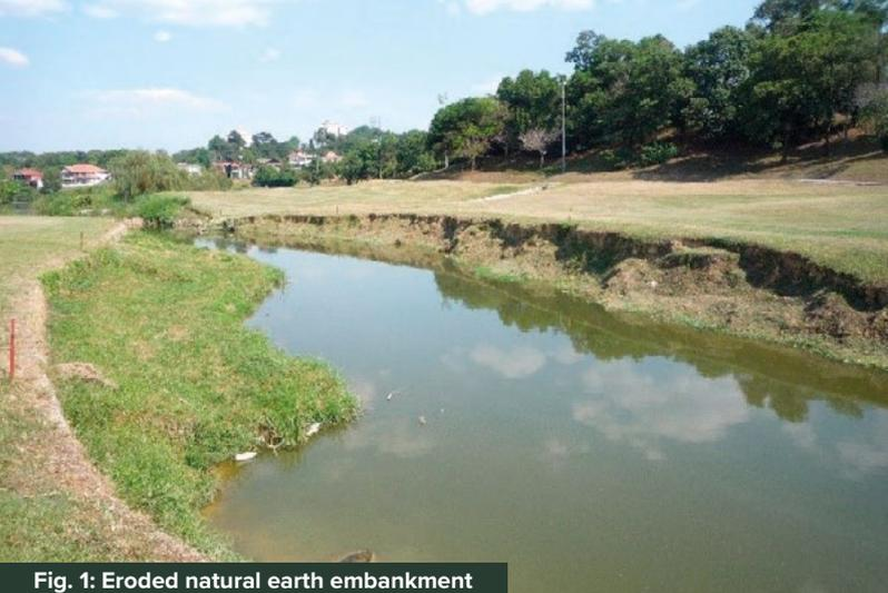
Fig. 1: Eroded natural earth embankment
