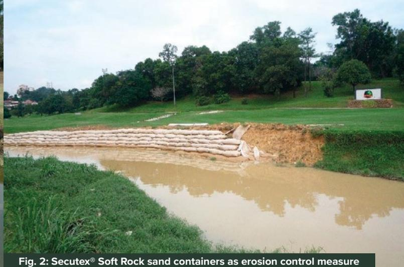
Fig. 2: Secutex® Soft Rock sand containers as erosion control measure
