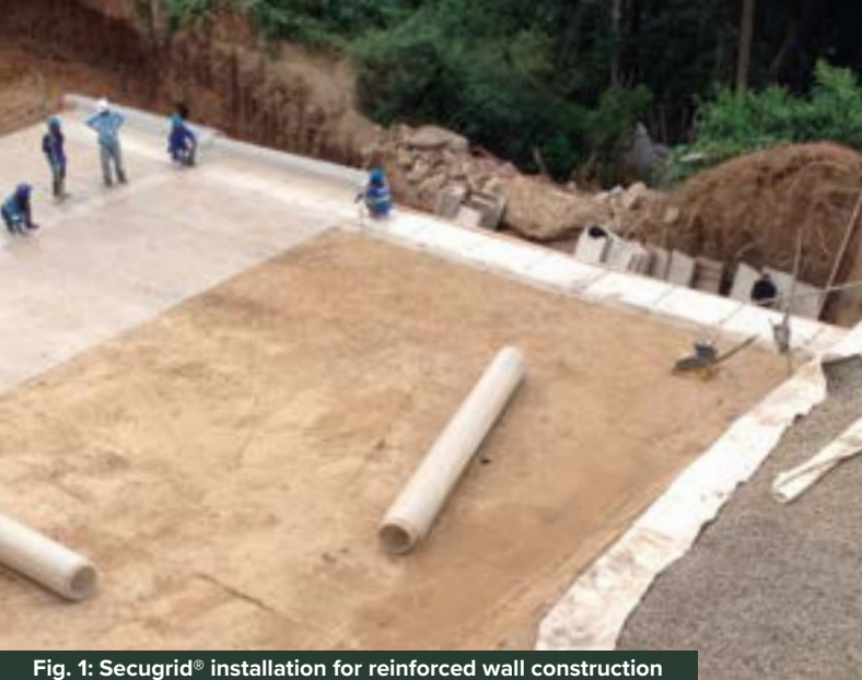
Fig. 1: Secugrid® installation for reinforced wall construction
