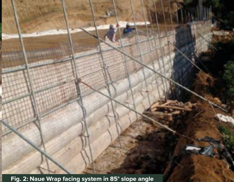
Fig. 2: Naue Wrap facing system in 85° slope angle
