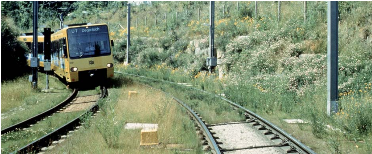
Fig. 1: City railway Stuttgart, Germany. Example of a greened up geogrid reinforced supporting structure (1990)
