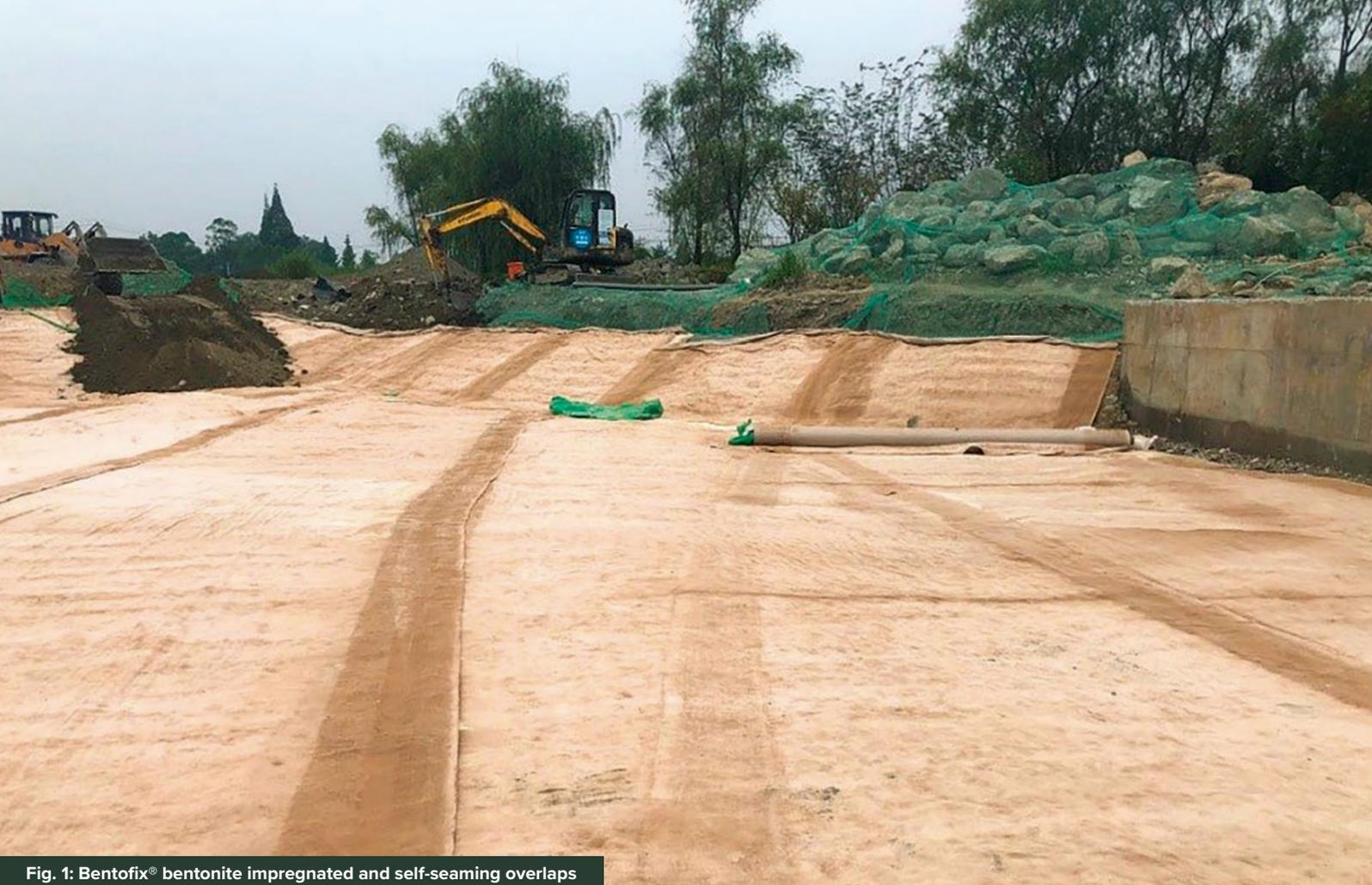
Fig. 1: Bentofix® bentonite impregnated and self-seaming overlaps
