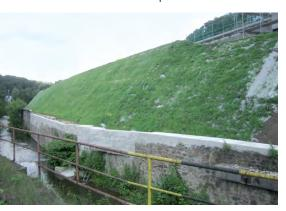
The NAUE NAIL system can provide temporary or permanent steep slope reinforcement. It is characterized by a high degree of flexibility, allowing for significant adaptation to project-specific requirements, site layouts and conditions while still providing a high-strength yet economical slope-reinforcement solution with natural, long-term vegetation cover.
