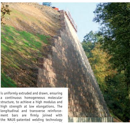
high strength at low elongations. The longitudinal and transverse reinforcement bars are firmly joined with the NAUE-patented welding technology to provide a structurally sound and stable geogrid for reinforcement applications. Secugrid® is used for base reinforcement, mechanically stabilised earth (MSE) wall construction including veneer stabilisation, the segmental re-
