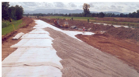
Fig. 3 Covering Bentofix® GCL with locally available fine gravel to ward off burrowing animals
