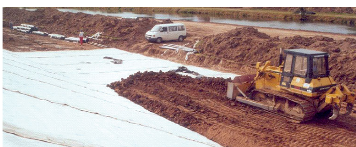
Fig. 5 Kinzig River levee reconstruction (2001)
