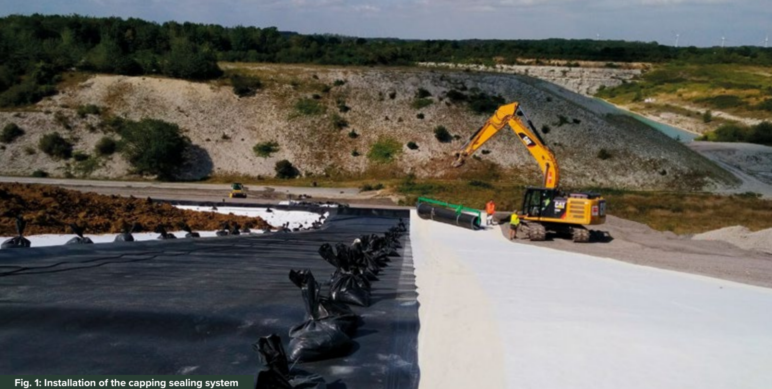
Fig. 1: Installation of the capping sealing system
