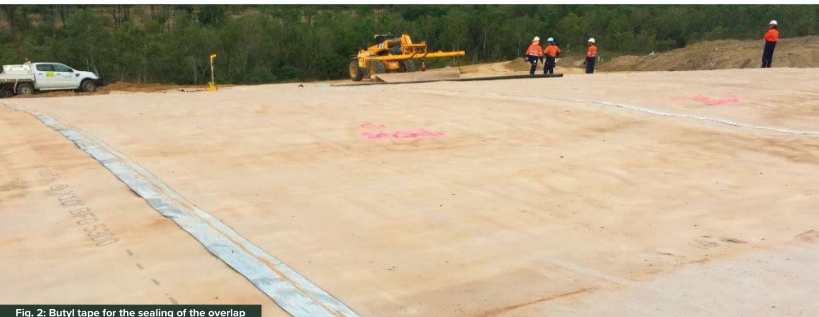
**Fig. 2: Butyl tape for the sealing of the overlap**
