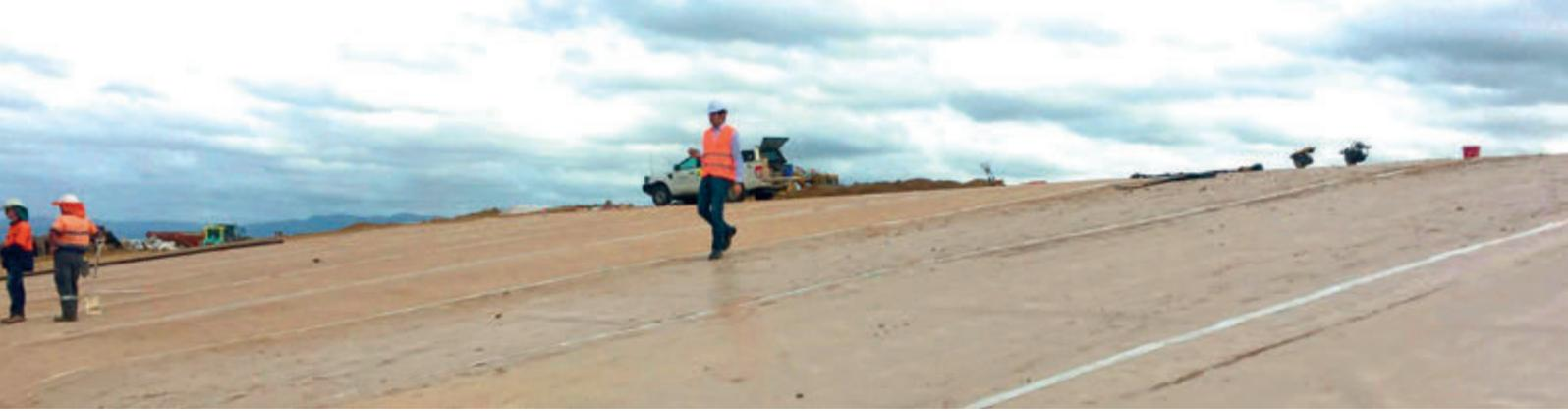
Fig. 1: Bentofix® as landfill capping system
