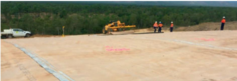
Fig. 2: Butyl tape for the sealing of the overlap
