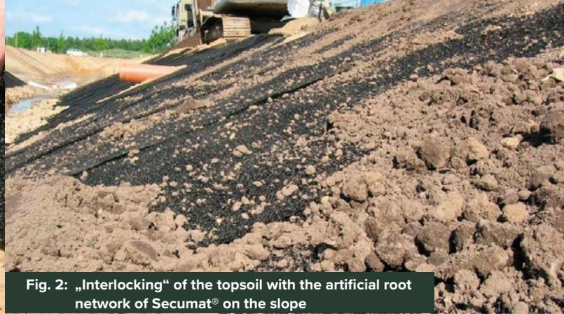
**Fig. 2: „Interlocking“ of the topsoil with the artificial root network of Secumat® on the slope**
