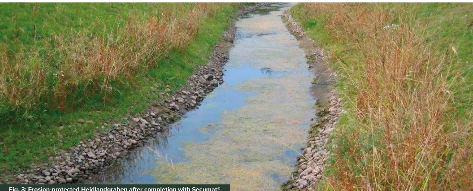
**Fig. 3: Erosion-protected Heidlandgraben after completion with Secumat®**
