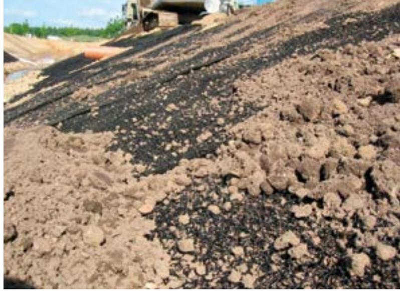
Fig. 2: „Interlocking“ of the topsoil with the artificial root network of Secumat® on the slope
