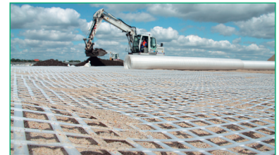
Figure 13 Secugrid® installation
