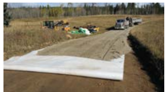
Figure 7: Combigrid® and Secugrid® installation
