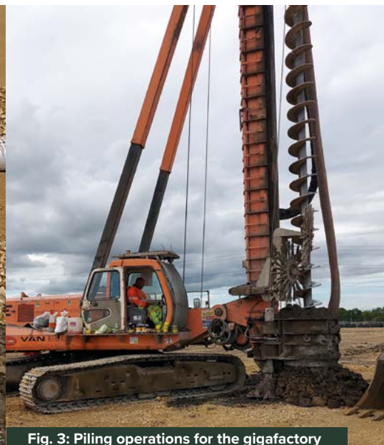
Fig. 3: Piling operations for the gigafactory
