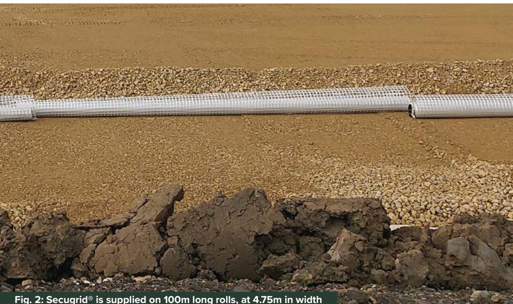
Fig. 2: Secugrid® is supplied on 100m long rolls, at 4.75m in width
