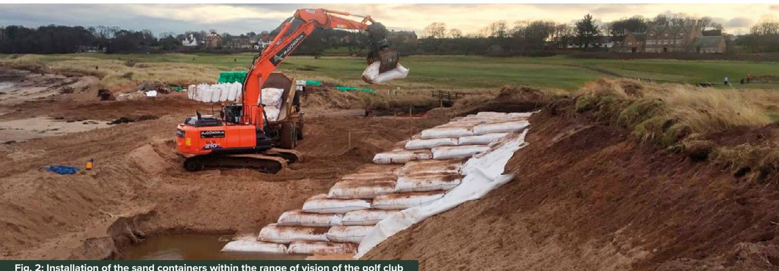
**Fig. 2: Installation of the sand containers within the range of vision of the golf club**
