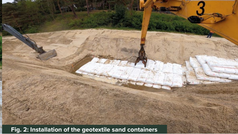
Fig. 2: Installation of the geotextile sand containers
