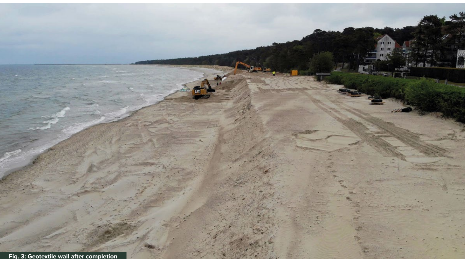
Fig. 3: Geotextile wall after completion
