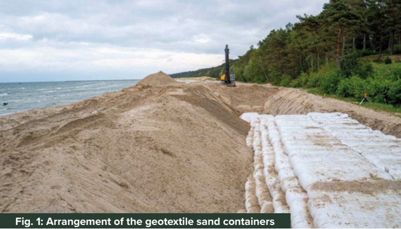
Fig. 1: Arrangement of the geotextile sand containers
