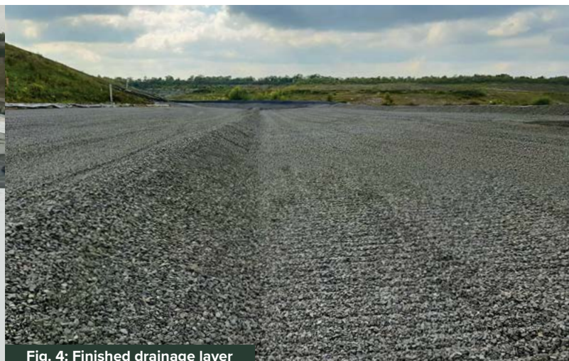
Fig. 4: Finished drainage layer
