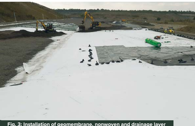
Fig. 3: Installation of geomembrane, nonwoven and drainage layer
