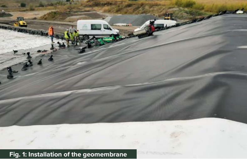
Fig. 1: Installation of the geomembrane
