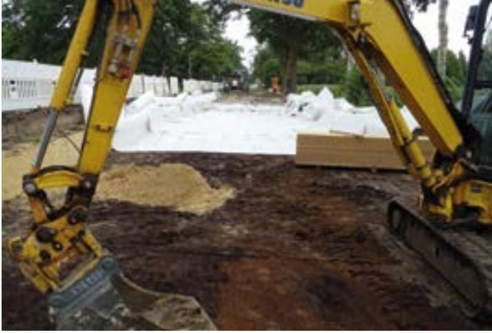
Fig. 1: Installation of Combigrid® as base reinforcement in the construction area
