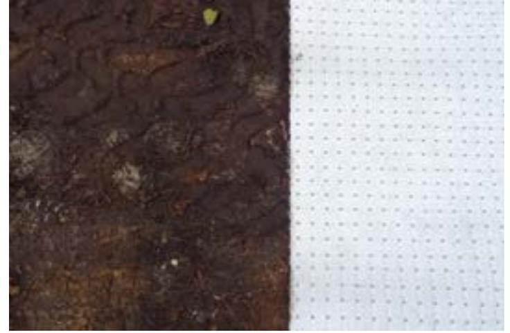
Fig. 2: Detail - Combigrid® on subsoil with low bearing capacity
