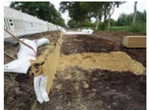
Fig. 3: Securing the natural gas pipeline in the lateral area
