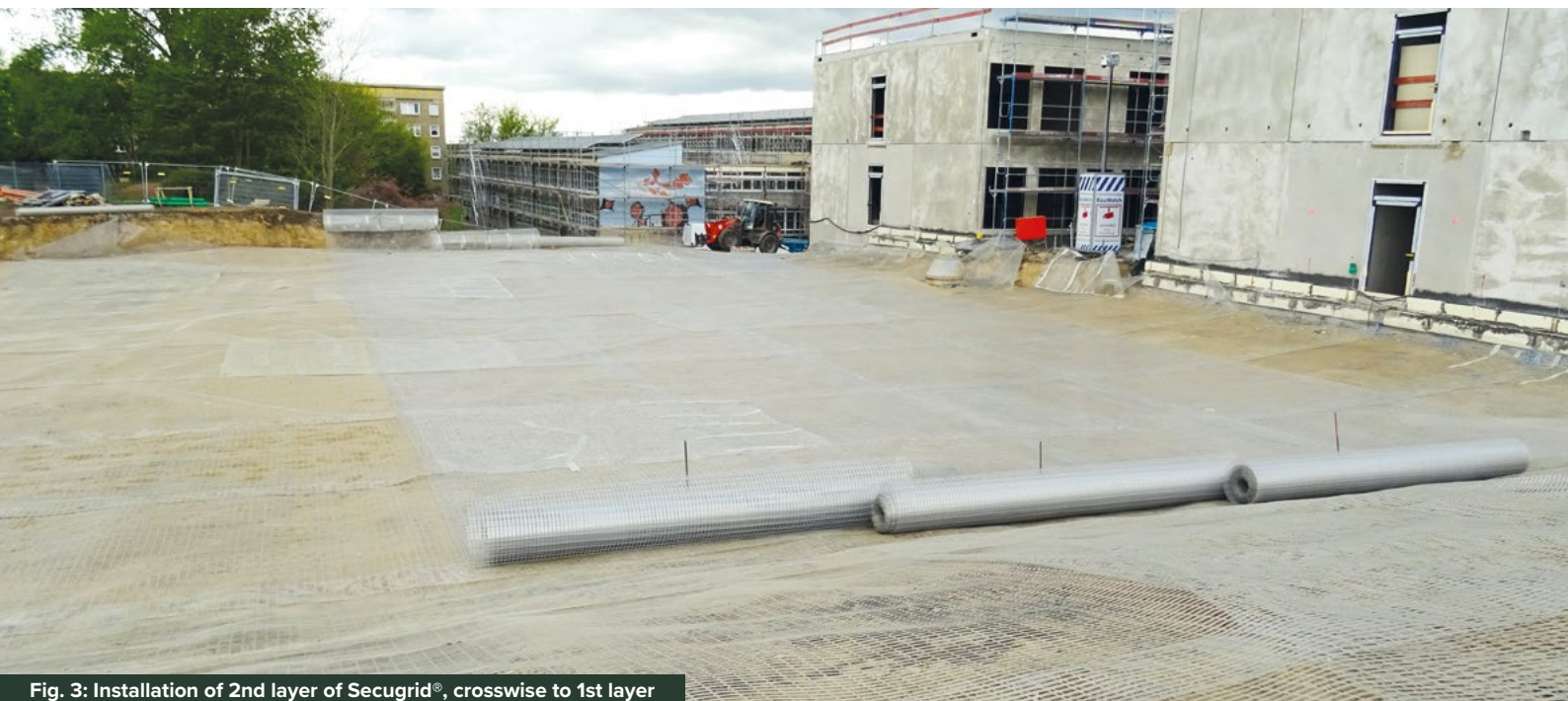
Fig. 3: Installation of 2nd layer of Secugrid®, crosswise to 1st layer
