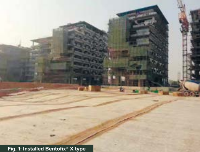
Fig. 1: Installed Bentofix® X type
