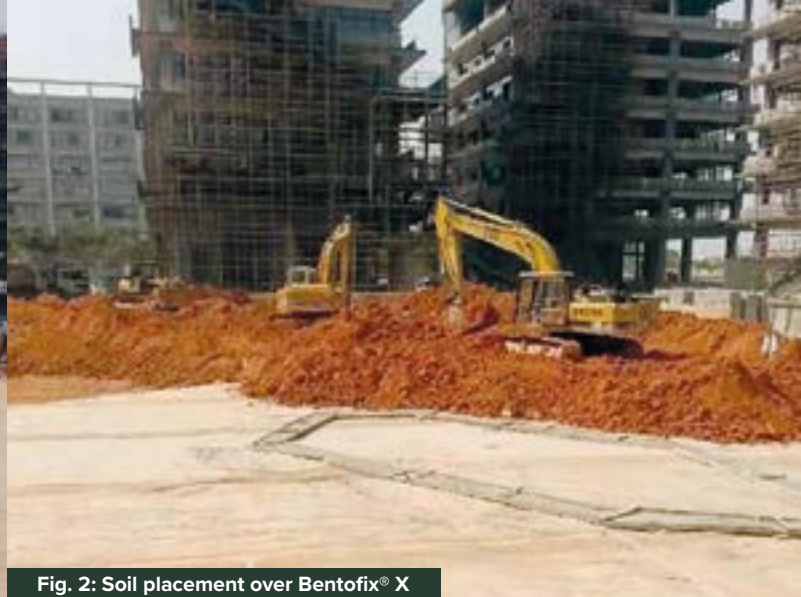
Fig. 2: Soil placement over Bentofix® X
