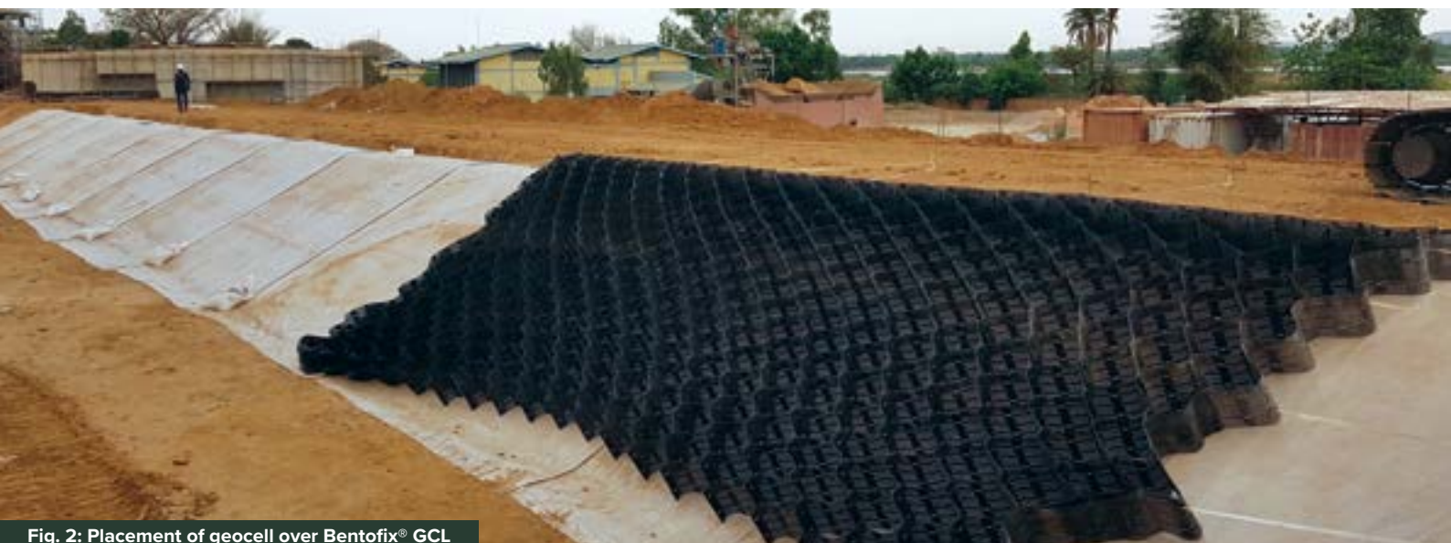
Fig. 2: Placement of geocell over Bentofix® GCL
