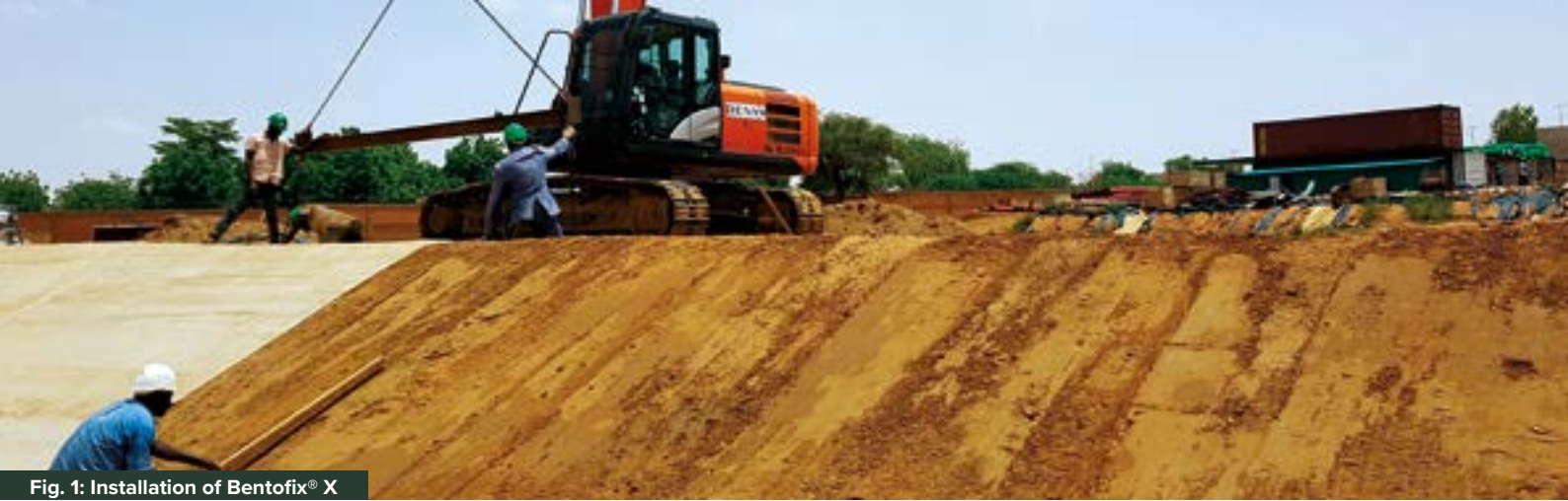
Fig. 1: Installation of Bentofix® X
