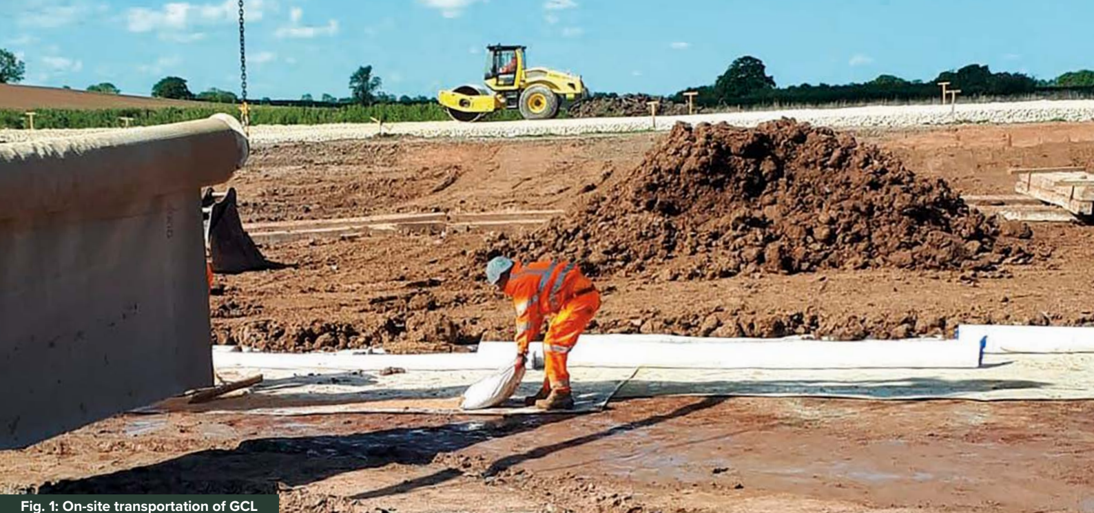
Fig. 1: On-site transportation of GCL
