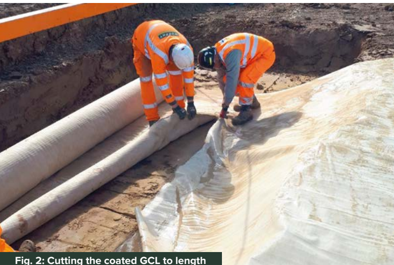
Fig. 2: Cutting the coated GCL to length
