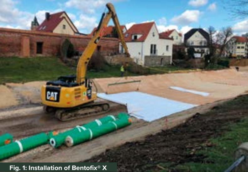
Fig. 1: Installation of Bentofix® X
