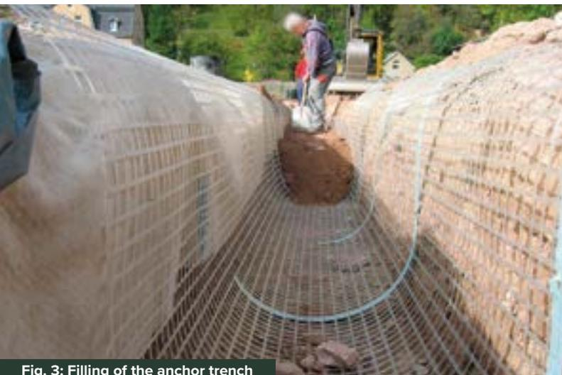
Fig. 3: Filling of the anchor trench
