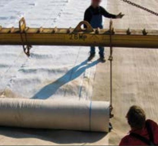
Fig. 1: Installation of Bentofix® with a spreader bar
