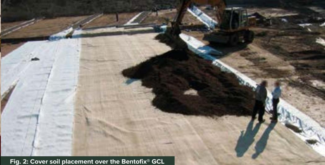
Fig. 2: Cover soil placement over the Bentofix® GCL
