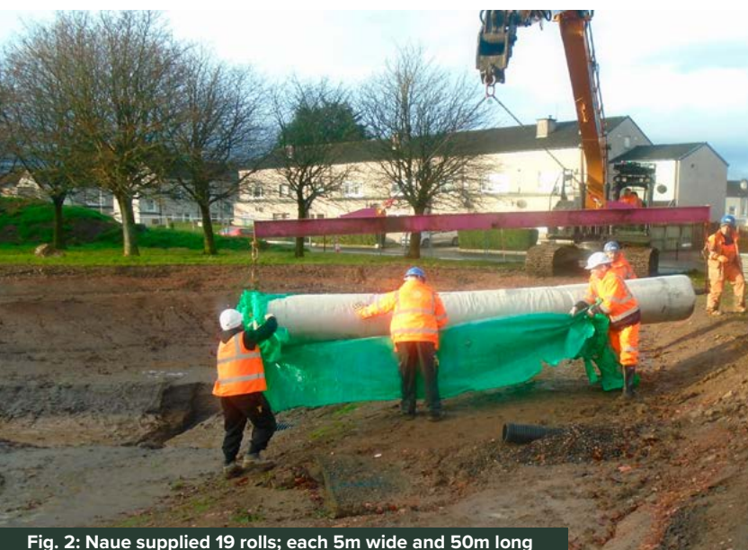
Fig. 2: Naue supplied 19 rolls; each 5m wide and 50m long
