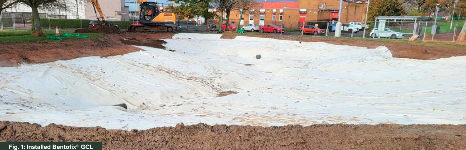
Fig. 1: Installed Bentofix® GCL
