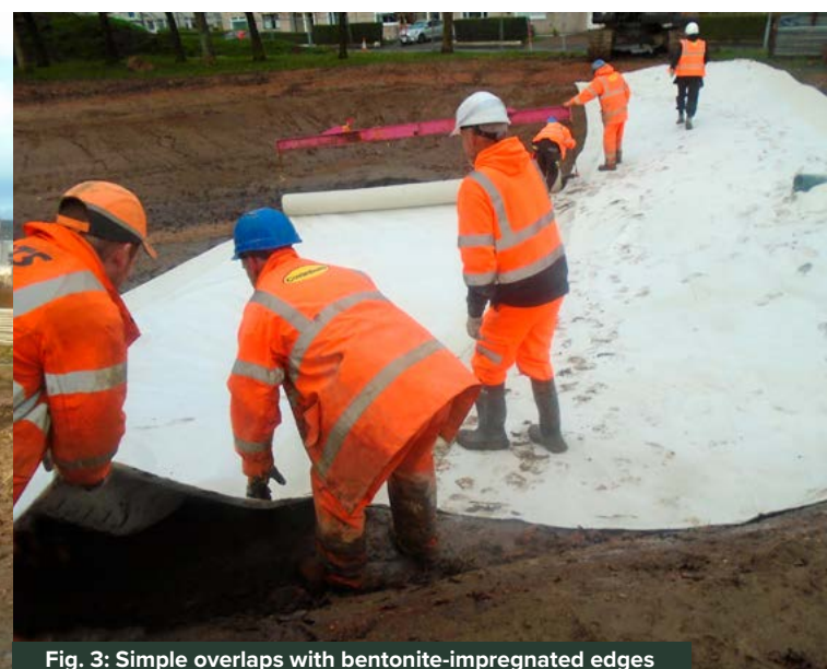
Fig. 3: Simple overlaps with bentonite-impregnated edges
