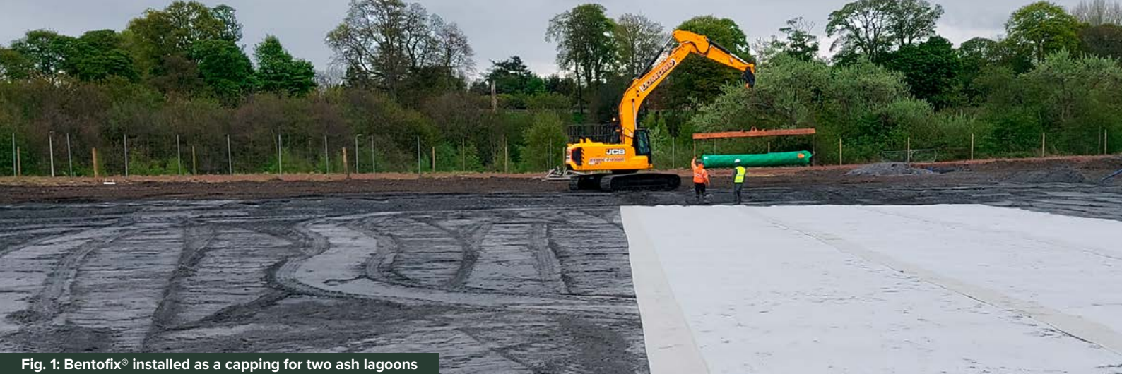
Fig. 1: Bentofix® installed as a capping for two ash lagoons
