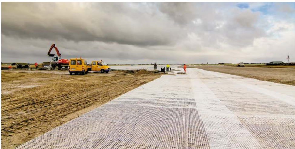
Figure 5: Large-scale installation of a Secugrid® stabilised and reinforced base course
