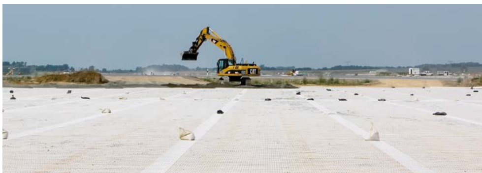
Figure 7: Installation of base course aggregate on top of Secugrid®
