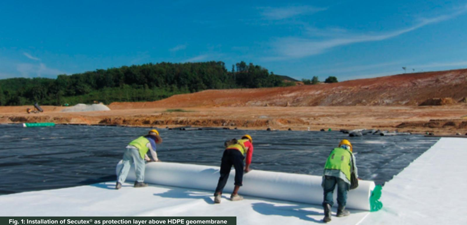
Fig. 1: Installation of Secutex® as protection layer above HDPE geomembrane
