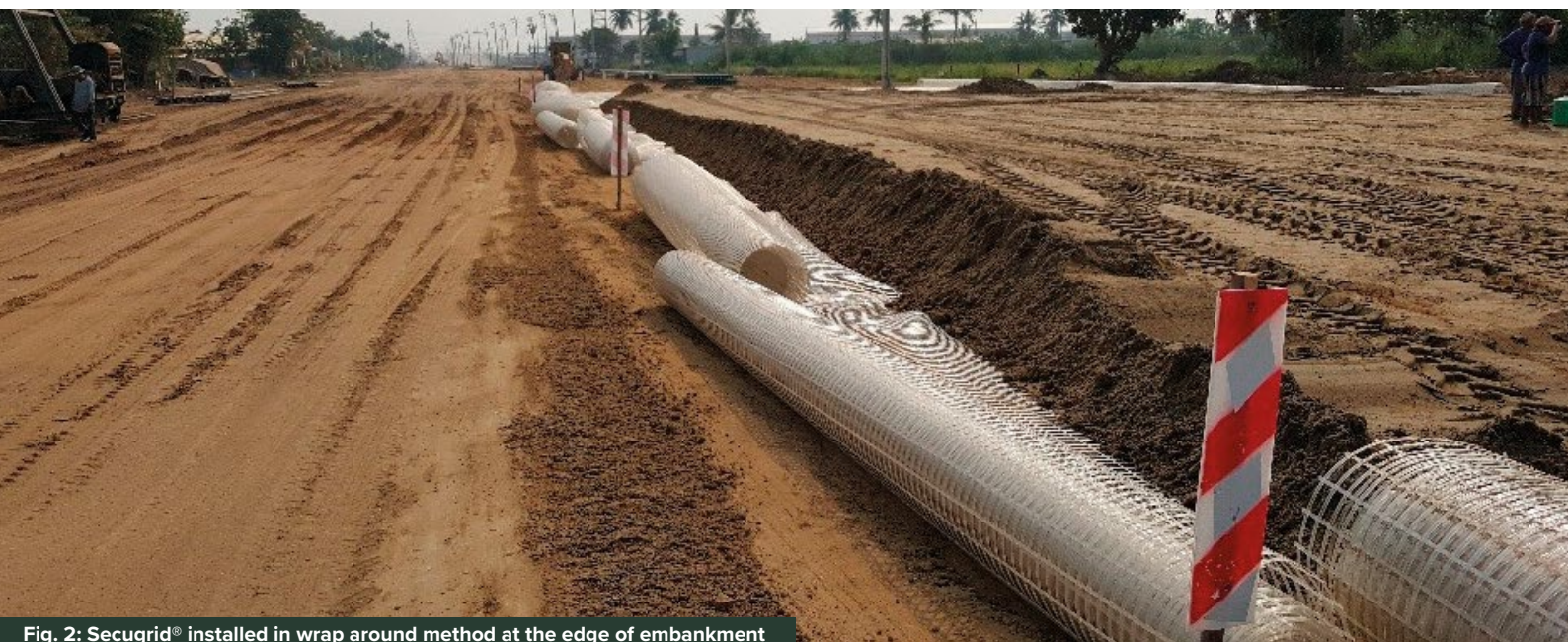
Fig. 2: Secugrid® installed in wrap around method at the edge of embankment
