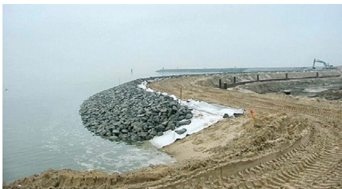
Figure 4: Revetment construction with Secutex® H
