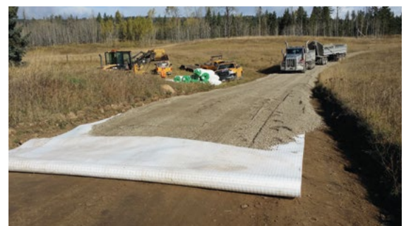
Figure 7: Combigrid® and Secugrid® installation
