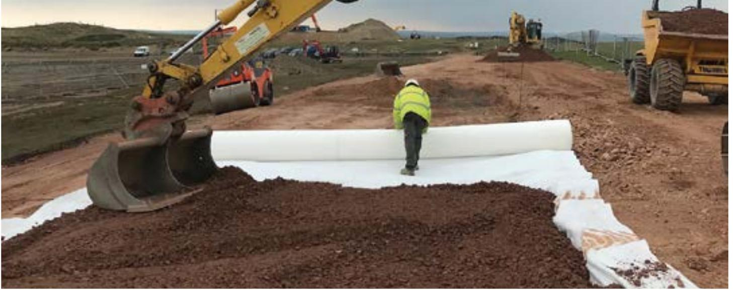
A layer of Secutex® Green 30G1 GRK 2 was also used on the embankment prior to installation of further Grasscrete™ paving.
