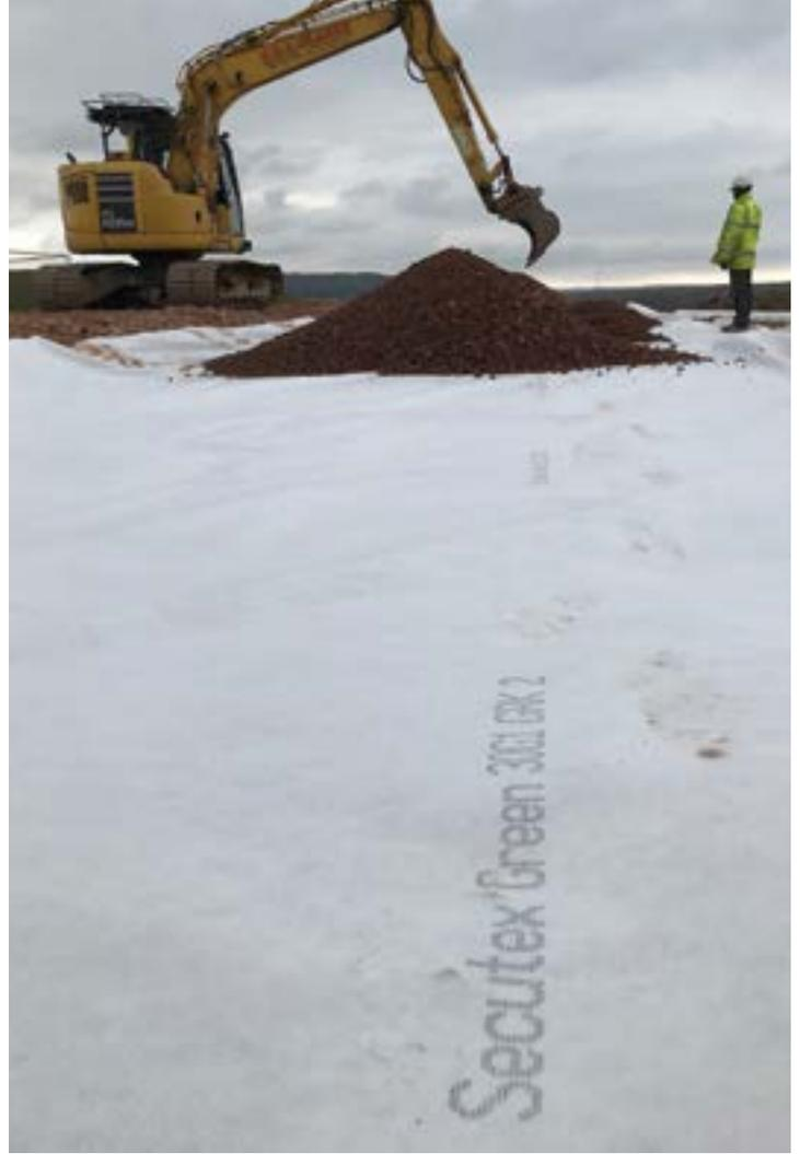
For the first time in the UK, a new and innovative biodegradable geotextile from NAUE Geosynthetics has been used in the construction of an elevated access road and car parking area for the Visitor Centre at Northam Burrows Country Park on the North Devon coast.
