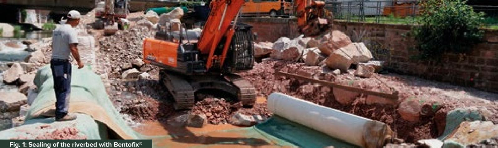
**Fig. 1: Sealing of the riverbed with Bentofix®**
