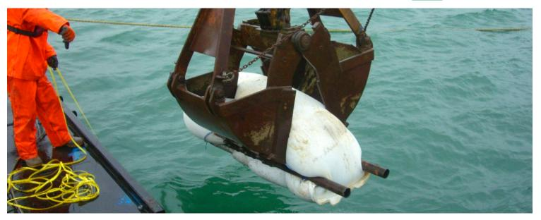
At ABP Port of Southampton's City Cruise Terminal, Naue geotextile sand containers have been installed to remediate scour holes in the harbour bottom and prevent further scour.
