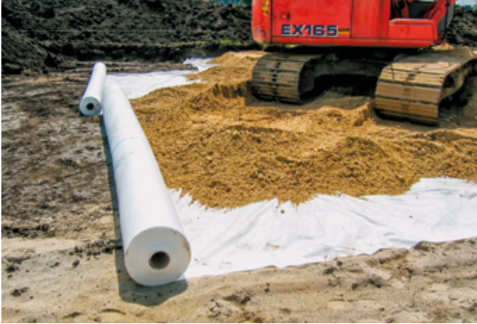
Figure 7: Secutex® as a separation layer - installation under heavy installation loads
