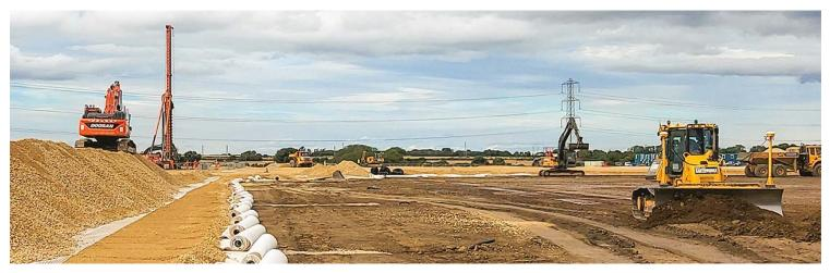
Naue have supplied Combigrid® and Secugrid® products for use in the construction of working platforms, to support piling and crane operations, during construction of a gigafactory which will span 50 hectares of land at the International Advanced Manufacturing Park (IAMP) in the north east of England, on the border between South Tyneside and Sunderland.
