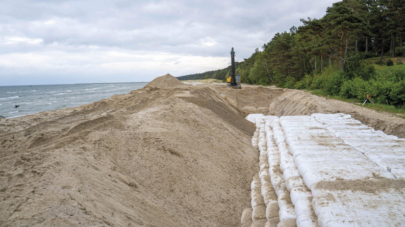
Fig. 1: Arrangement of the geotextile sand containers
