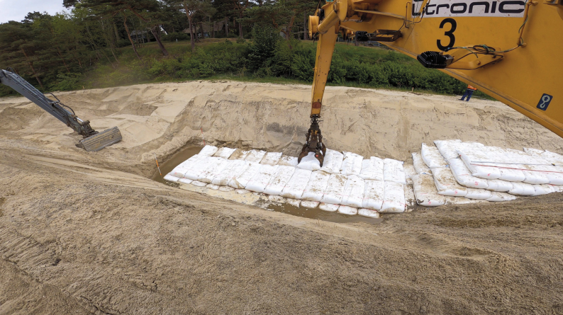
Fig. 2: Installation of the geotextile sand containers
