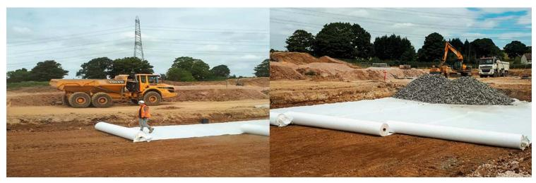
Naue's Combigrid® and Secugrid® products have been used success-fully to significantly improve the bearing capacity of the sub-base prior to construction commencing on site infrastructure for Lancaster University's new £14m Health Innovation Campus.
