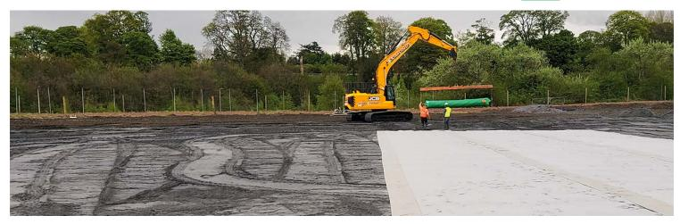
The ash lagoons at Levenhall Links, on the outskirts of Musselburgh, in Scotland, were constructed in the 1960s on land which had been reclaimed from the Forth estuary. Created to accommodate spoil from Scottish Power's coal-fired Cockenzie Power Station, which ceased operation in 2013, waste fly ash was mixed with water to form a slurry and then transported from the plant, through a network of pipes, to be deposited in the lagoons.
