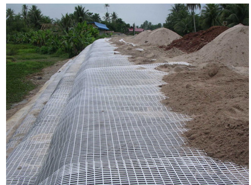
'Wrap-around' of Secugrid®
