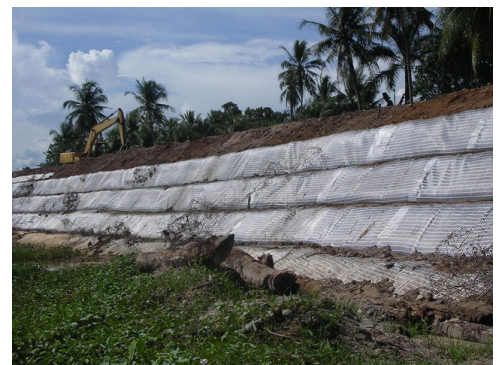
Layer spacing 1,0 m; Height 5,0 m
